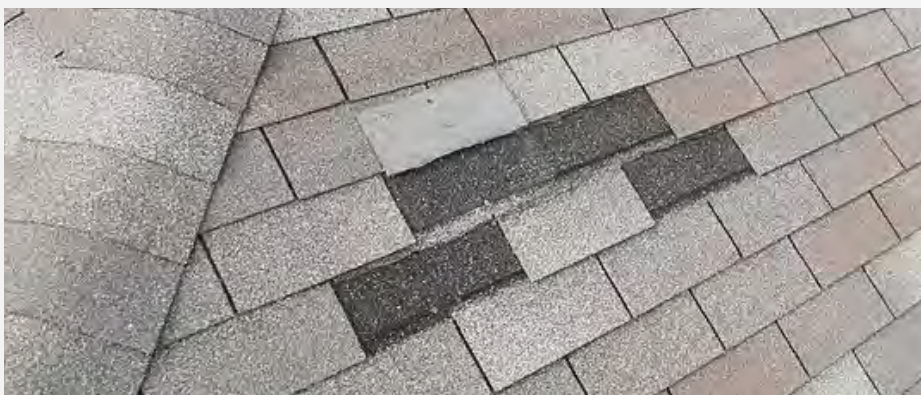
MISSING SHINGLES
